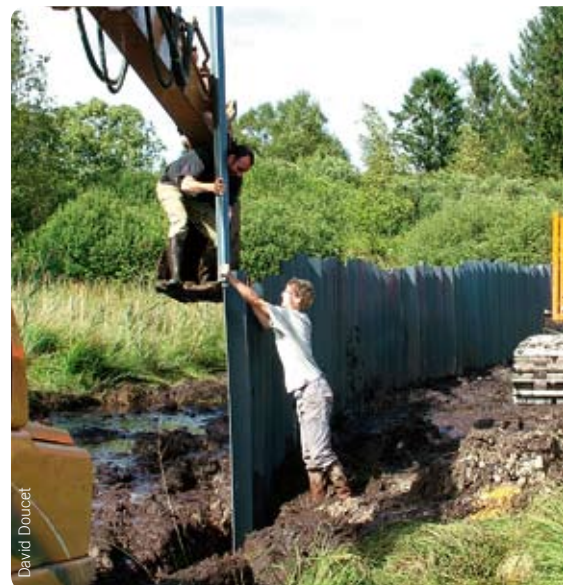
Construction of a dam with PVC sheet piles
